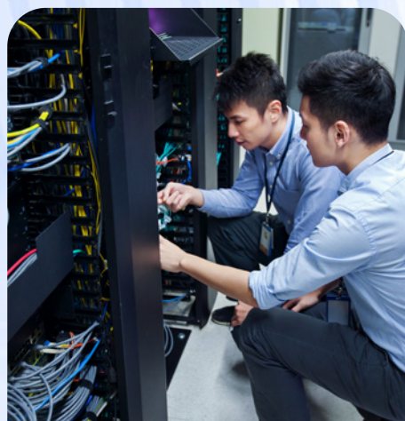
Cable Installation and Maintenance
