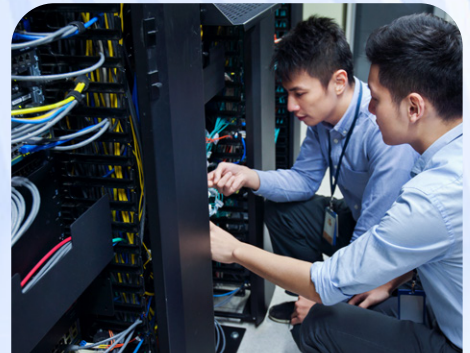
Cable Installation and Maintenance
